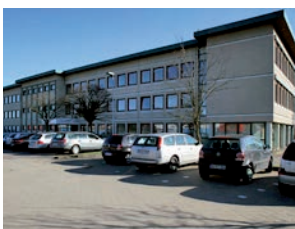
Hamburg industrial facility
